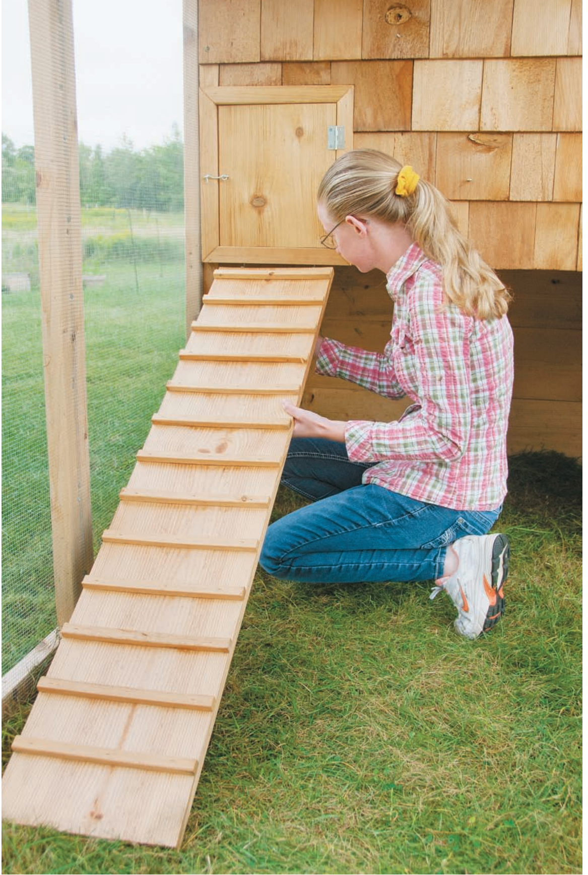
Now it's time to install the chicken ladder. The slats provide chickens with a way to grip the ladder and climb up.
