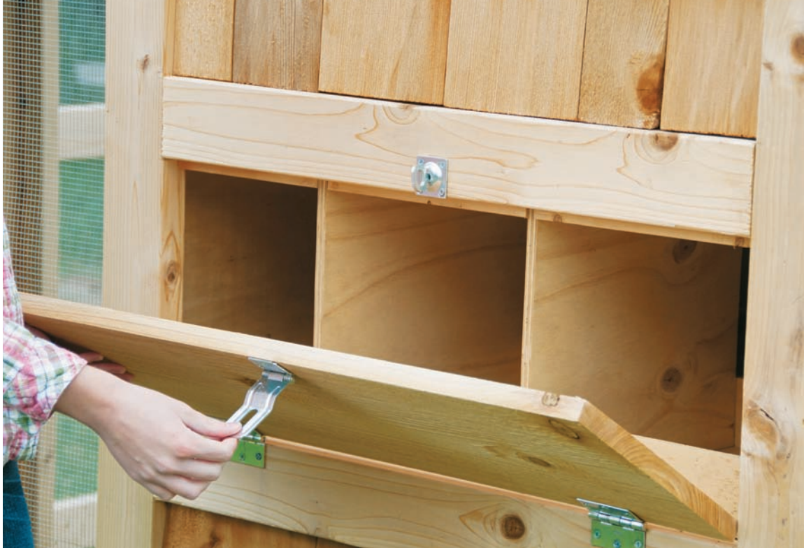
The egg collection door allows access to the nest boxes without having to go inside the coop.
