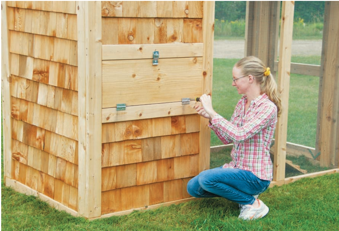
The cleanout door is identical to the egg collecting door and allows you to clean the inside of the coop from the outside. Handy!
