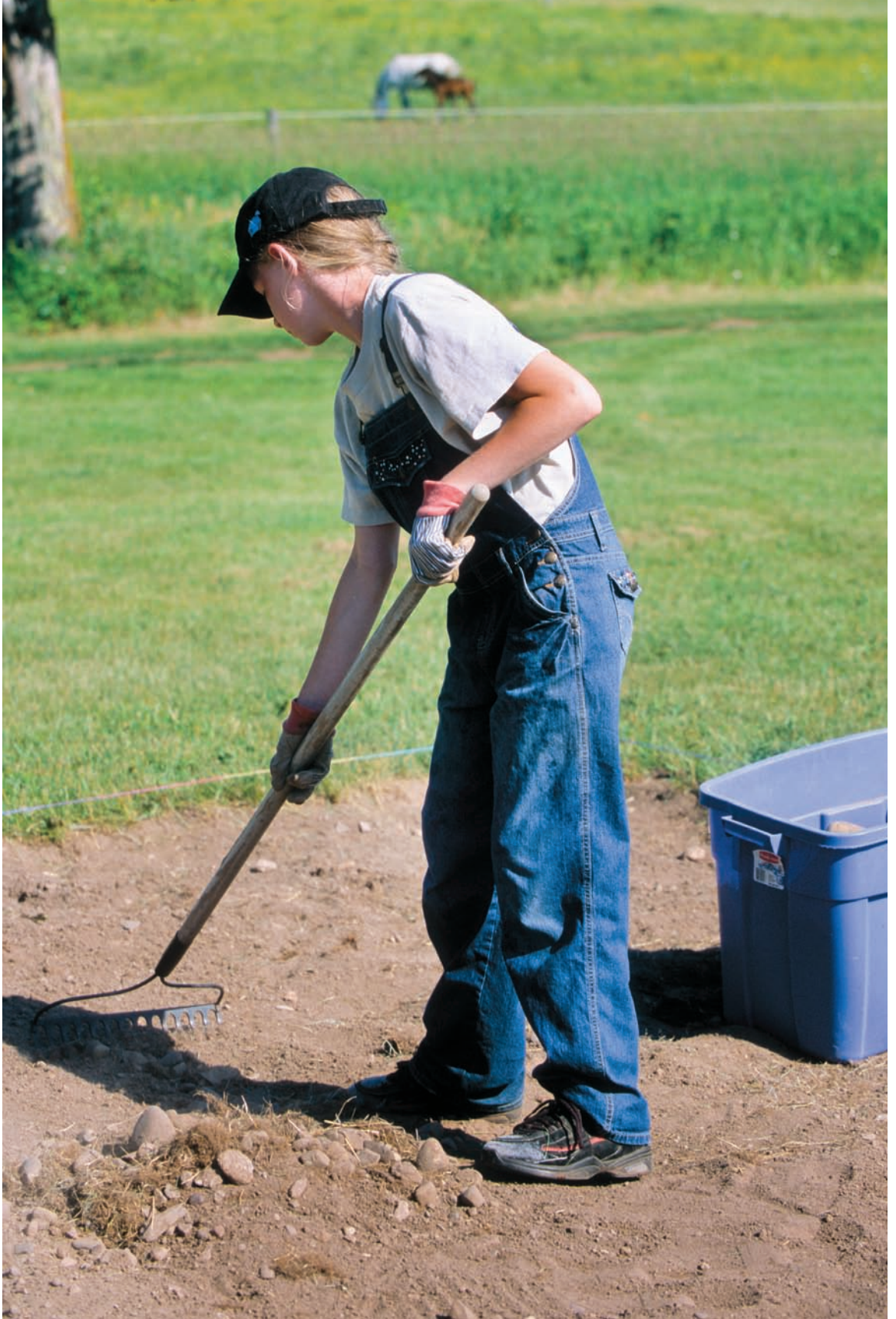
Preparing a site for your coop might entail some groundwork if your coop is going to be a permanent structure.
