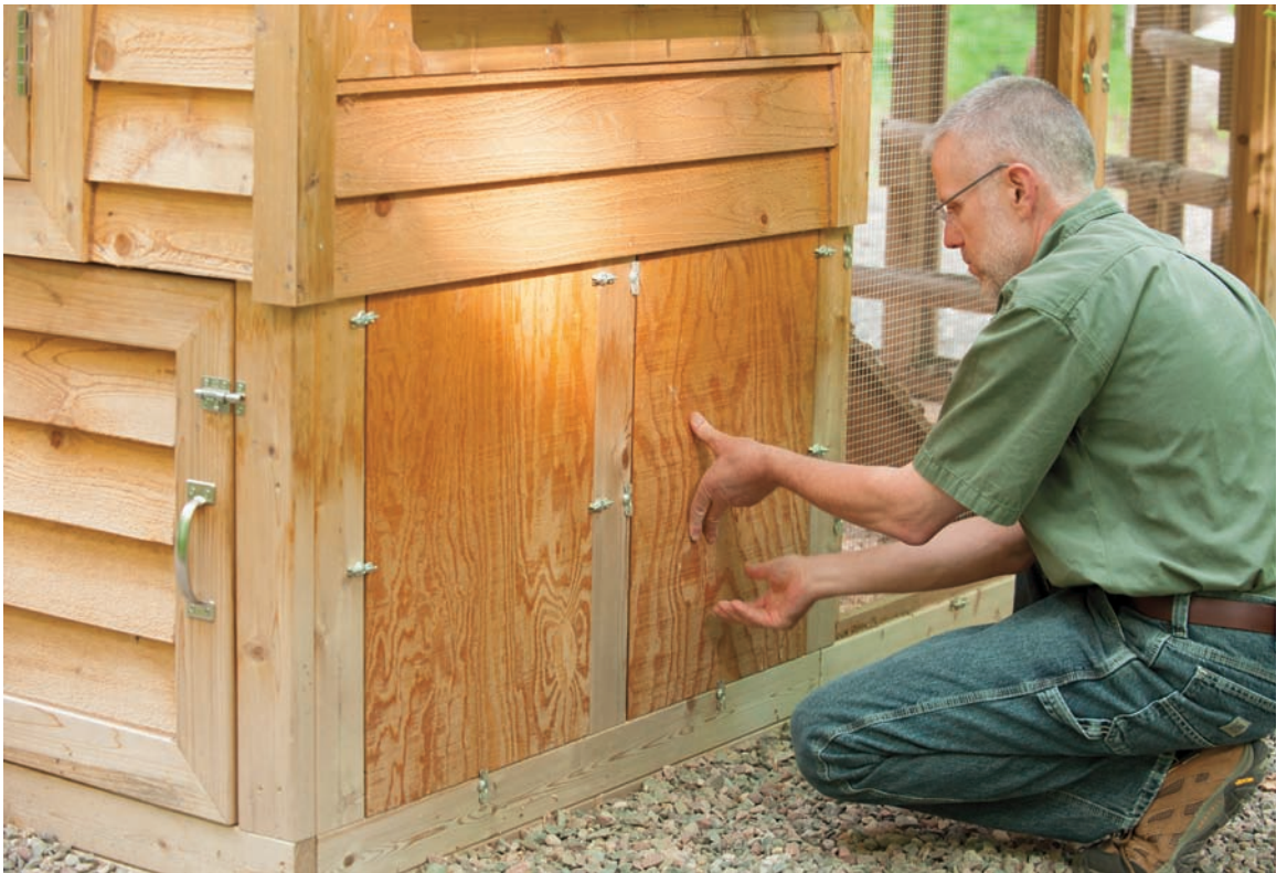
You can winterize your coop by adding wooden inserts to your run. They provide wind and rain protection to your hens and keep the coop and run a bit warmer during those frigid days of winter.
