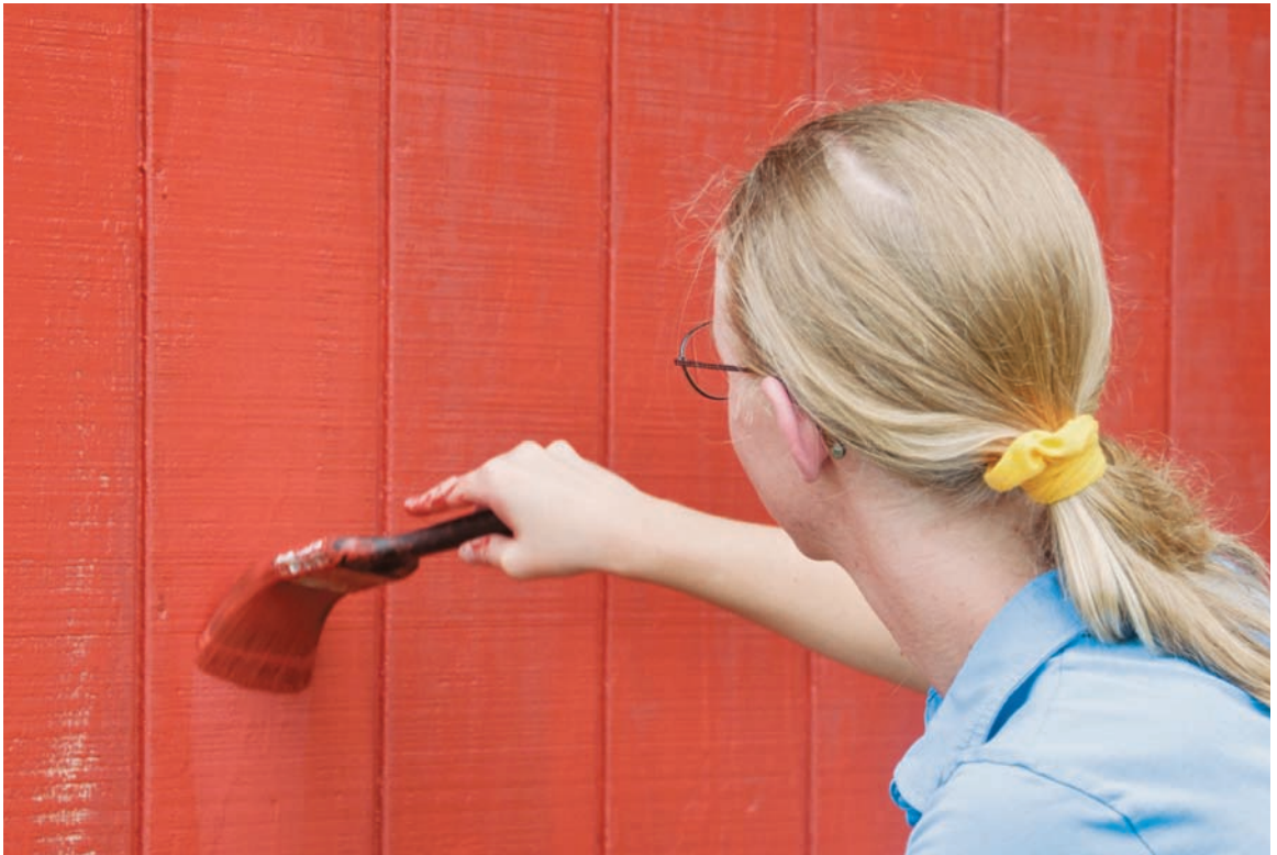
T1-11 is another option for the walls of your coop. It weighs less, but needs to be painted for protection from the elements.
