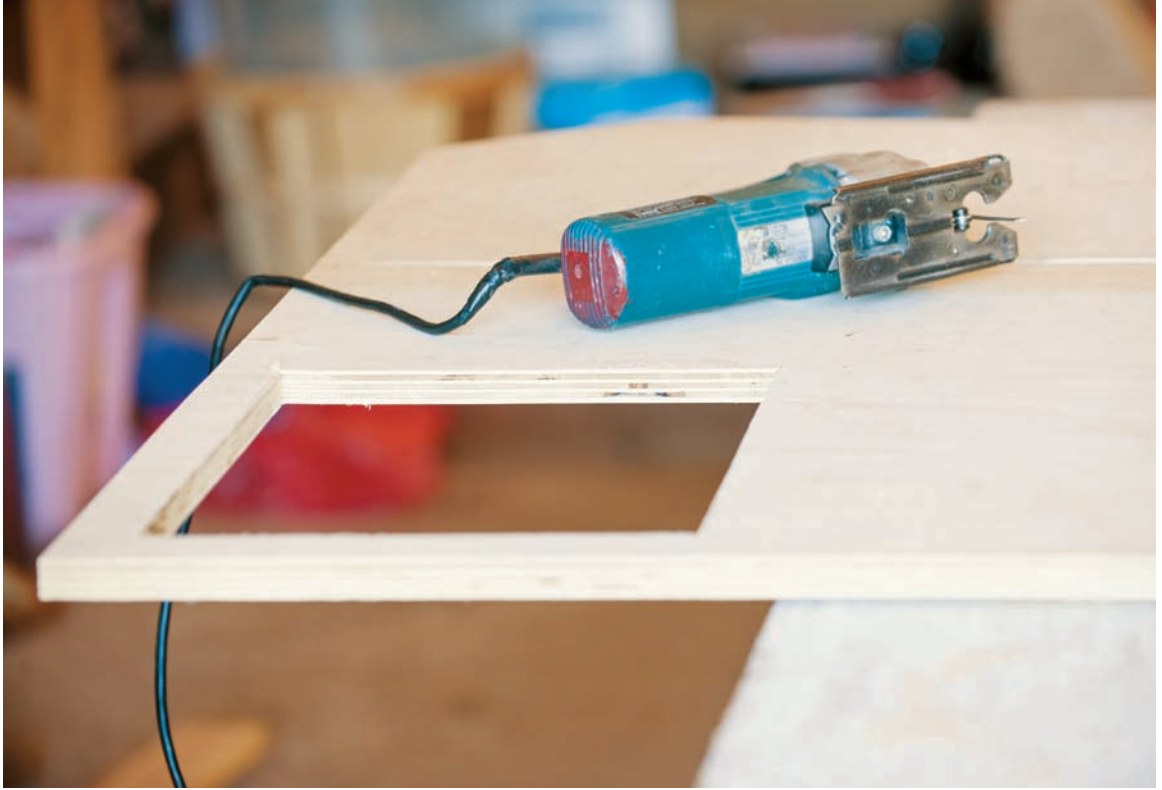
The finished doorway opening. Use a jigsaw to make precise cuts.
