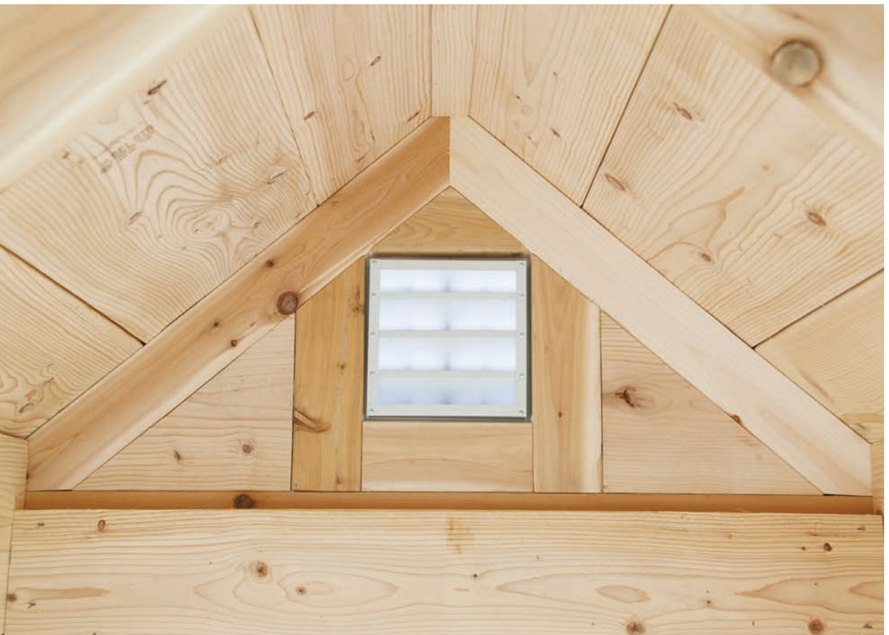
This is what the gable vent area will look like from the inside of the coop when it is completed. The 8 × 8-inch vent provides additional ventilation.
