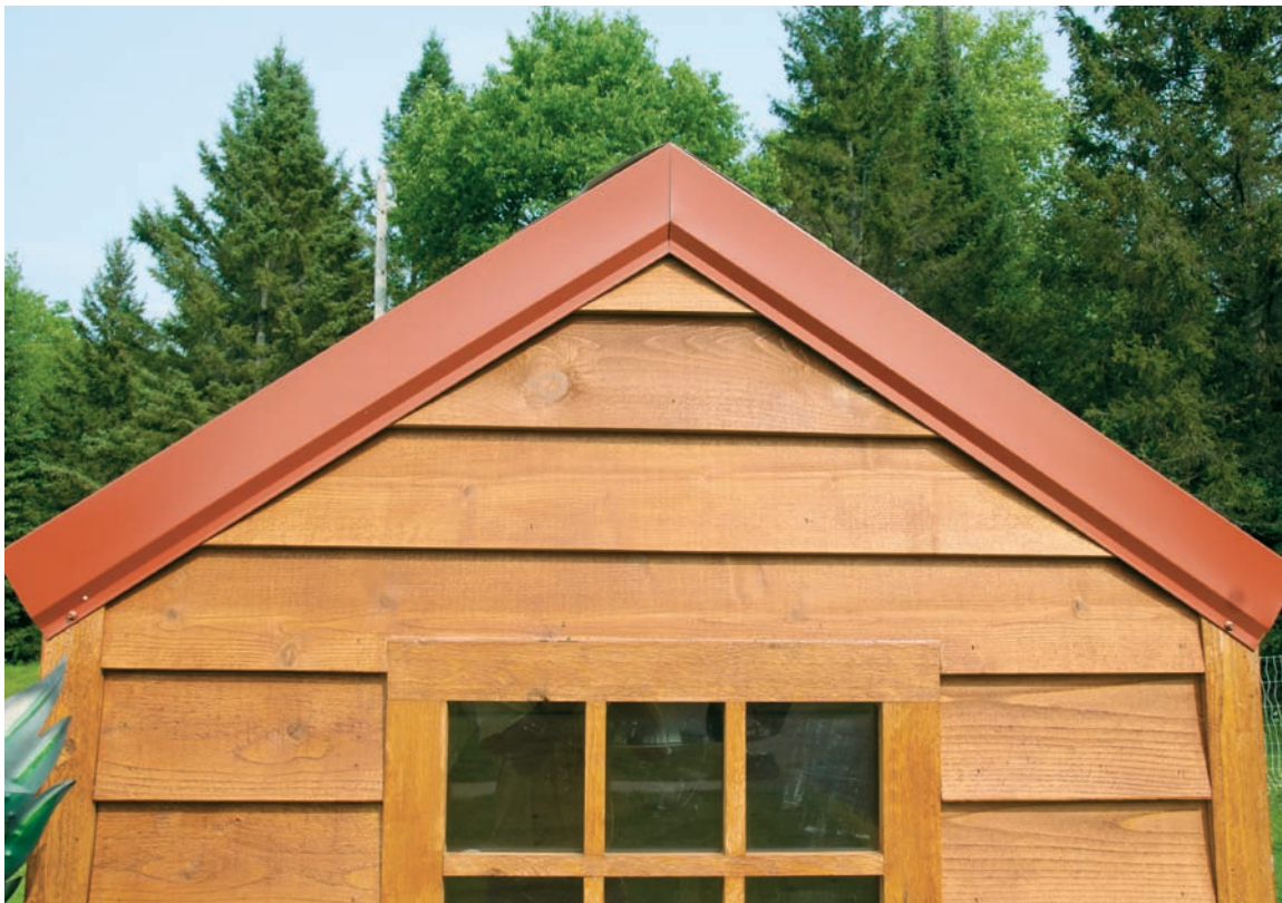
A gable roof is a common roof style for most houses and many chicken coops.
