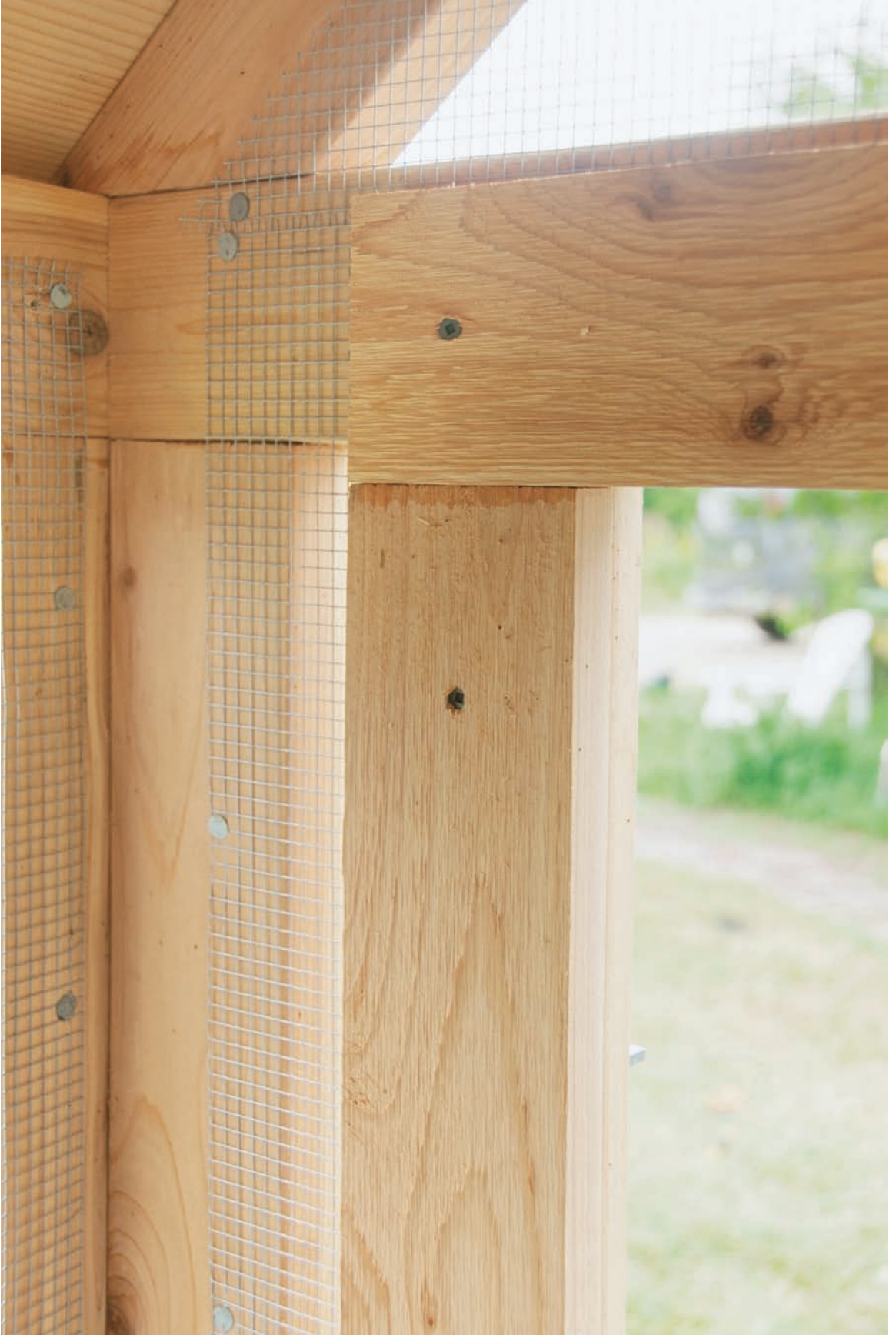
A simple doorstop just inside the coop will prevent the door from swinging too far inside.
