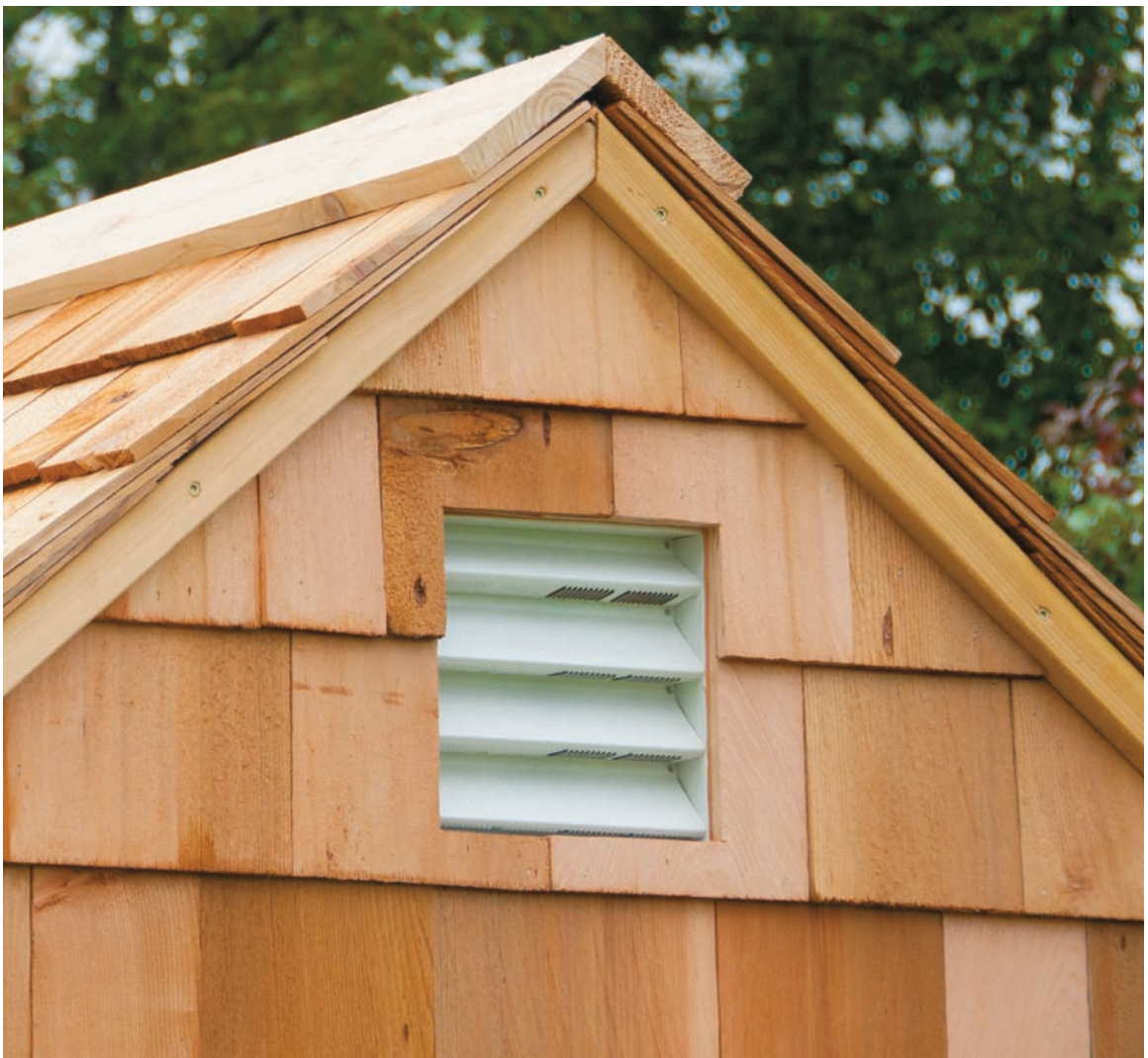
Adding a simple vent to your coop allows additional ventilation. Vents are easy to install and effectively keep out unwelcome guests.
