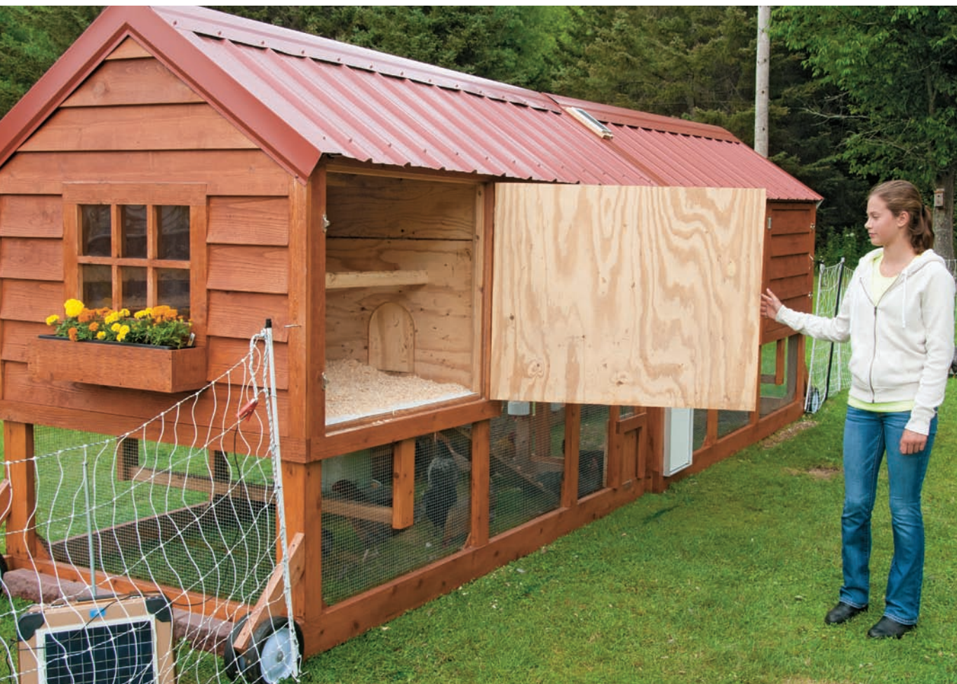
The large cleanout door on this coop makes accessing its interior easy, which makes cleanup less of a chore.
