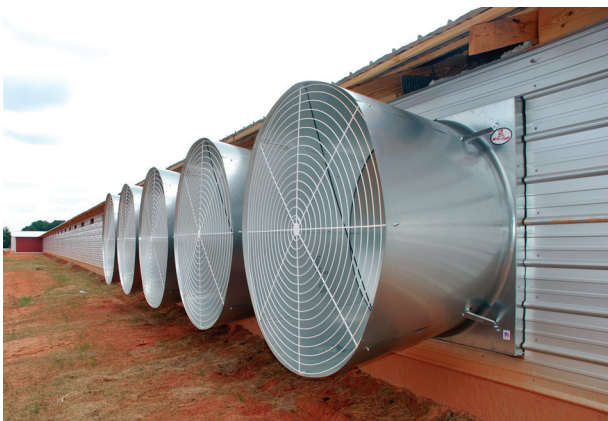
Figure 17.10 Exhaust fans moving air through a tunnel house. (Photo courtesy of Michael Czarick, University of Georgia Cooperative Extension Service)
