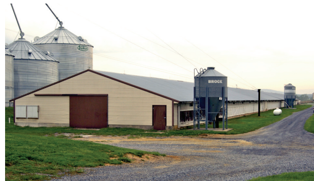
Figure 17.16 Curtain poultry house showing augering of feed to the poultry. (Source: USDA NRCS)
