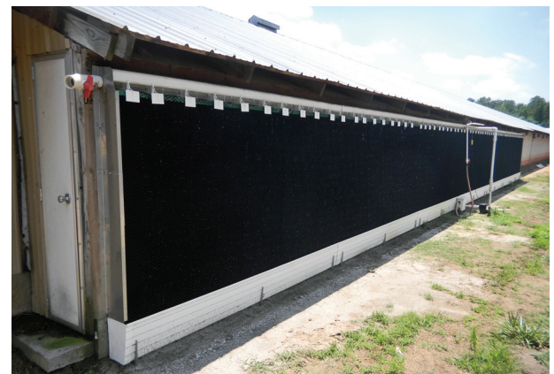
Figure 17.11 Cooling pads at air inlets in a tunnel house. The cooling pads reduce air temperatures experienced by the birds. (Photo courtesy of Michael Czarick, University of Georgia Cooperative Extension Service)
