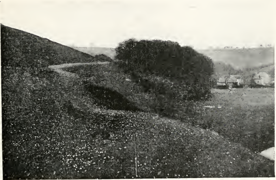
XX.—VIEW OF THE SAME ROADWAY BUT LOOKING IN THE OPPOSITE DIRECTION.
