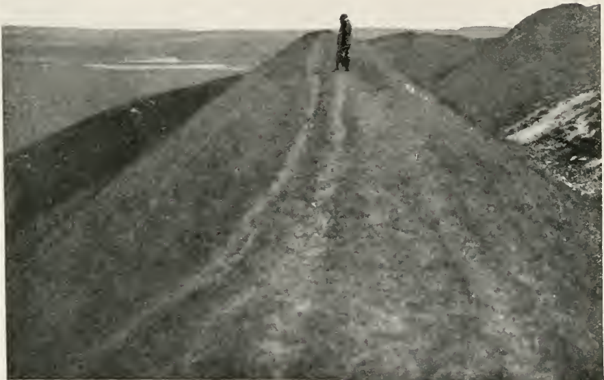
XVI.—VIEW FROM SUMMIT OF ONE OF THE SURROUNDING EMBANKMENTS AT MAIDEN CASTLE.
