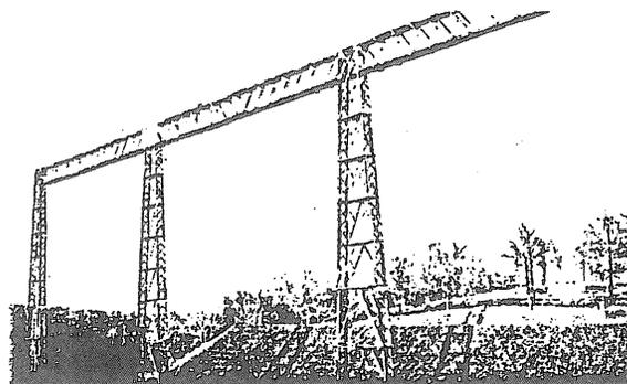
FIG. 3—The University of Illinois radio telescope. The focal line array, 155 feet above the 100-by-600-foot parabolic reflector, is visible below the wooden truss
