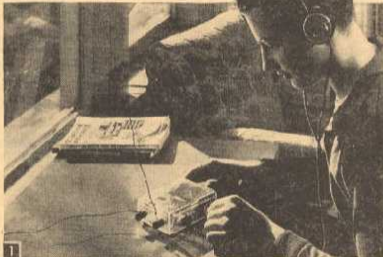
Testing the completed receiver, under (1) sunlight and (2) a 100 watt lamp. Direct sunlight naturally gives you much stronger reception.
