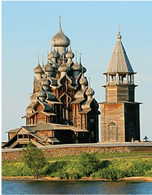
Figure 1.9 Listed as a UNESCO World Heritage Site, this church in Kizhi, Russia, is constructed entirely out of wood using the log building technique [1].
