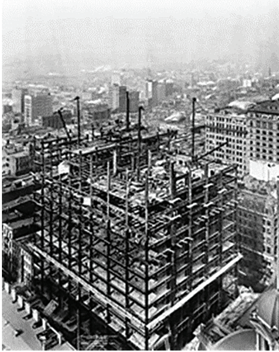
Figure 1.12 Woolworth Building under construction in 1912 [1].
